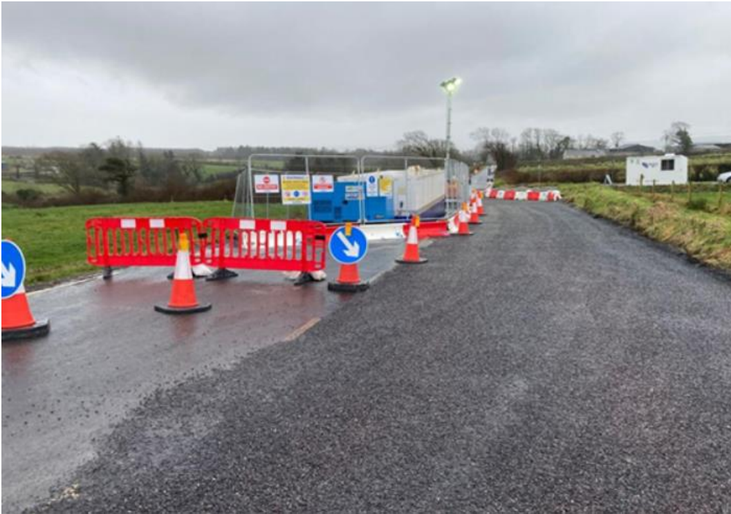
Figure 0.6: Operational Joint Bay with Passing Bay (on the Kilpaddoge Knockanure 220kV UGC Project, Co. Kerry – refer to Section 2.2.3 of the Volume 2A Planning Report)
